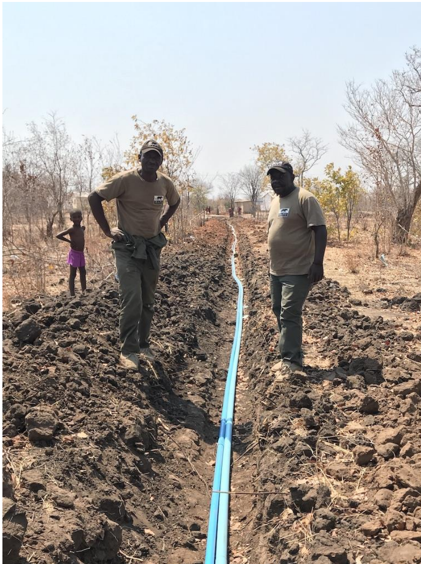
Fig. 15. Bongi and Muno checking for leaks before covering up trench.
