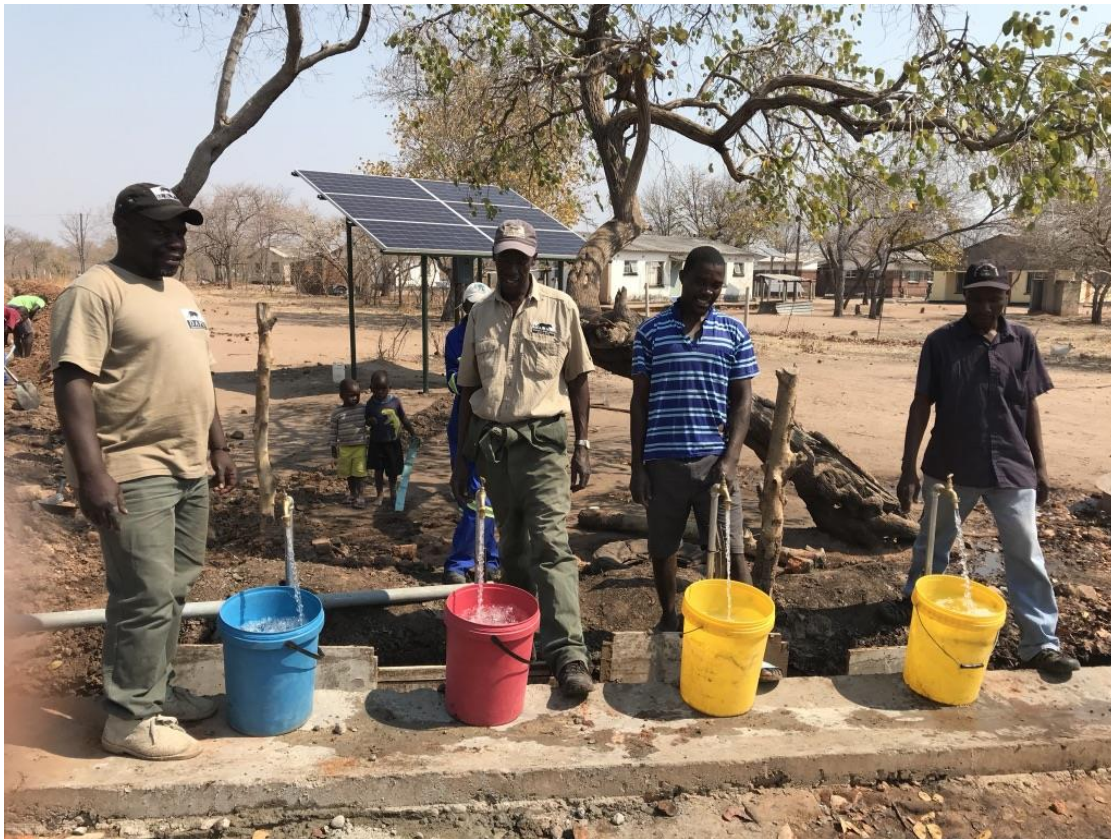
Fig. 17. It took 20 seconds to fill 4 x buckets (80 liters).
